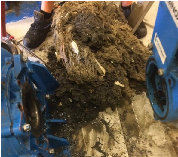
Figur 88 Tilstopping pumpe.
