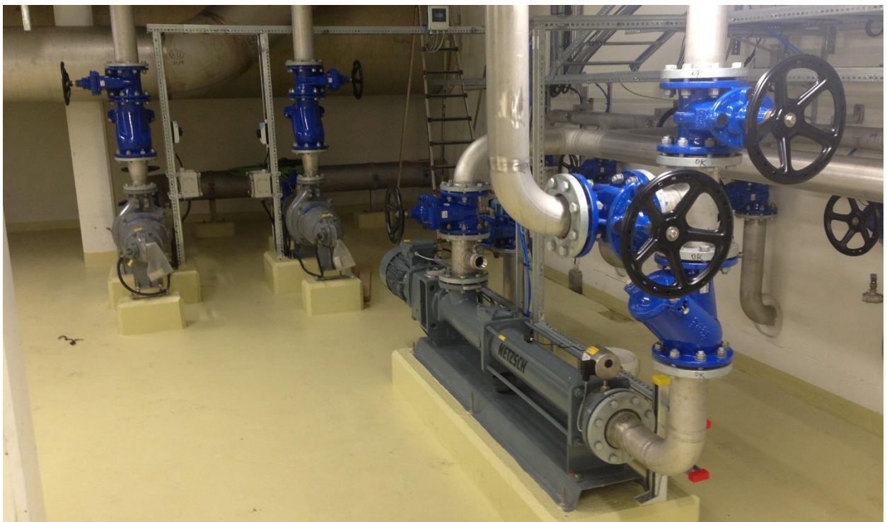
Figur 17 Odderøya rensanlegg – nye slampumper.
